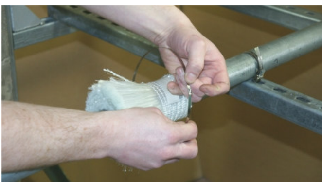
Use the stainless steel cable tie supplied or wire to prevent the fabric unrolling in the event of a fire
