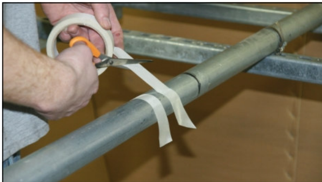
Pre-cut some short lengths of self adhesive tape to aid fixing, apply a length to the Brushseal then adhere to the penetration ensuring the bristles are aligned with the mark and then start the wrapping process
