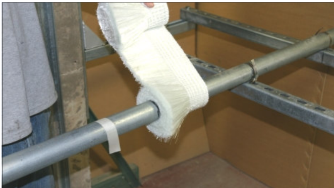
Wrap to a minimum of 5 layers and cut the seal fabric as shown then secure the seal with the self adhesive tape.
