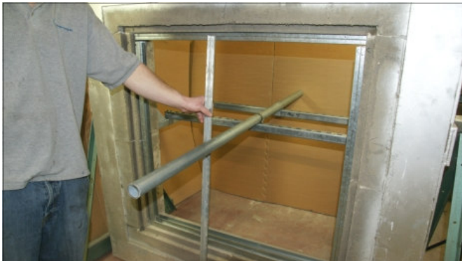
Using a straight edge mark the penetration where it will meet the fire barrier as shown above
